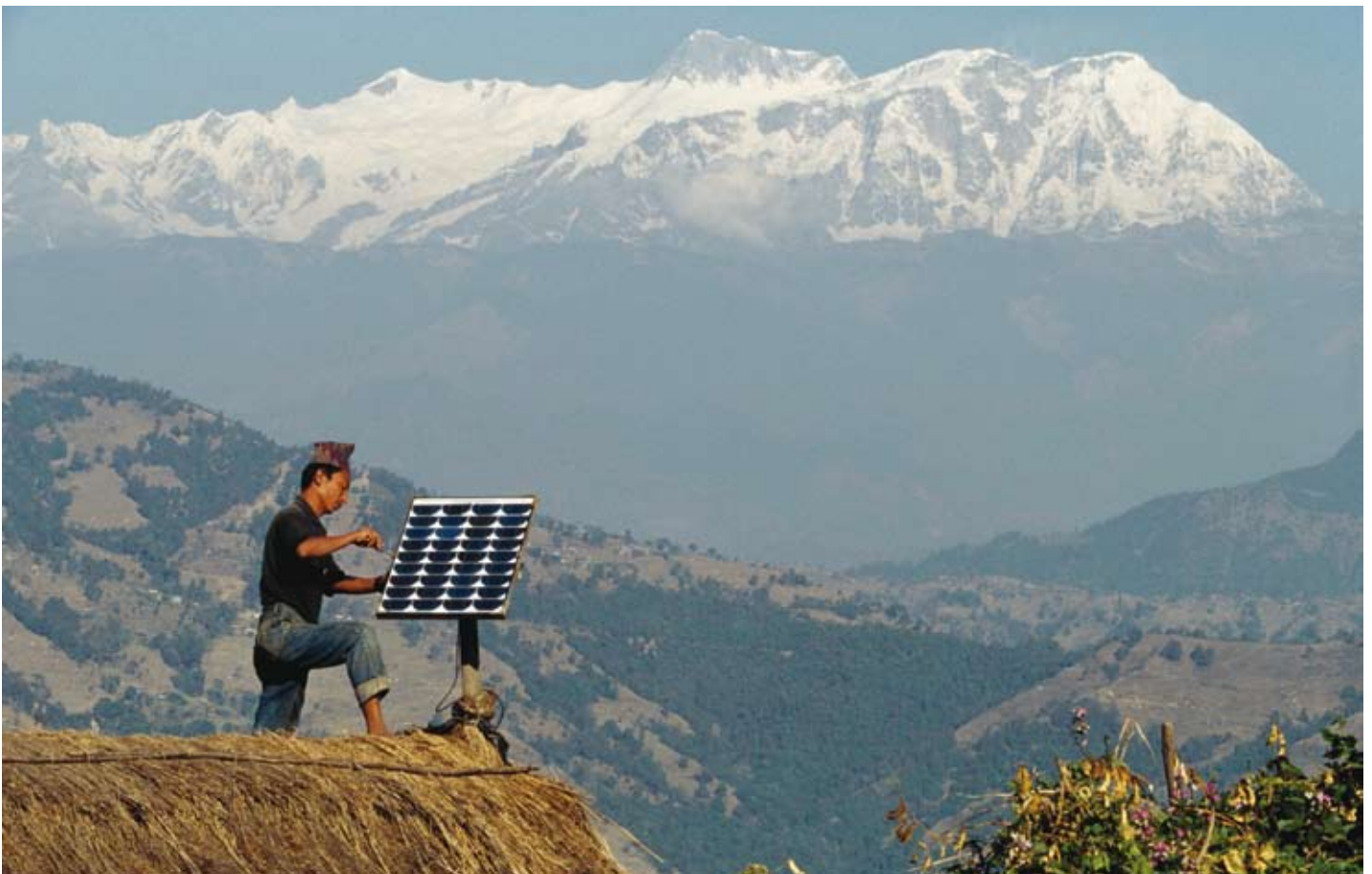
A Lotus Energy technician installs a solar panel in Nepal
