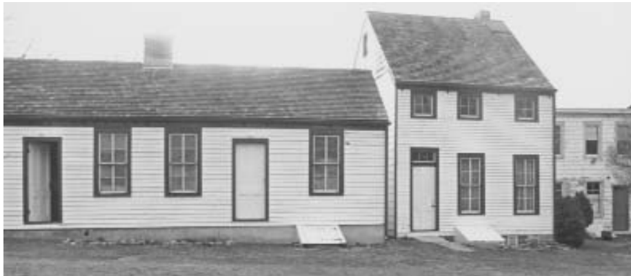
East elevations of three historic homes in Historic Weeksville, a nineteenth-century African-American community in Brooklyn. Currently managed by the Society for the Preservation of Weeksville and Bedford-Stuyvesant History, Weeksville was rediscovered in 1968 when its four remaining dwellings were spotted from the air.
