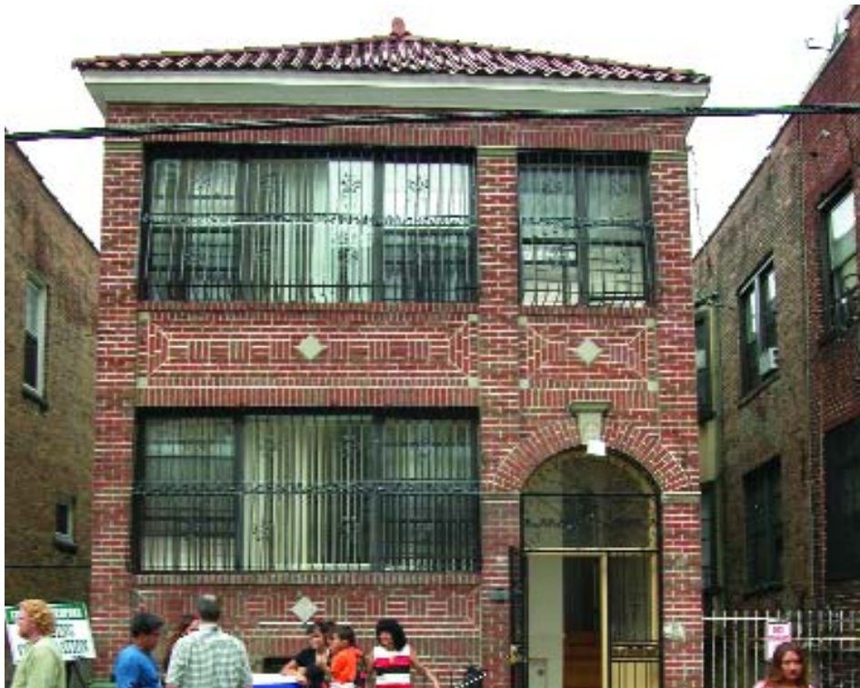
This home, located in the northwest section of the Bronx, was redeveloped from an uninhabitable shell through HPD's Neighborhood Homes Program in collaboration with the Enterprise Foundation and Fordham Bedford Housing Corporation. It is a three-family home with one owner unit and two rental units.
