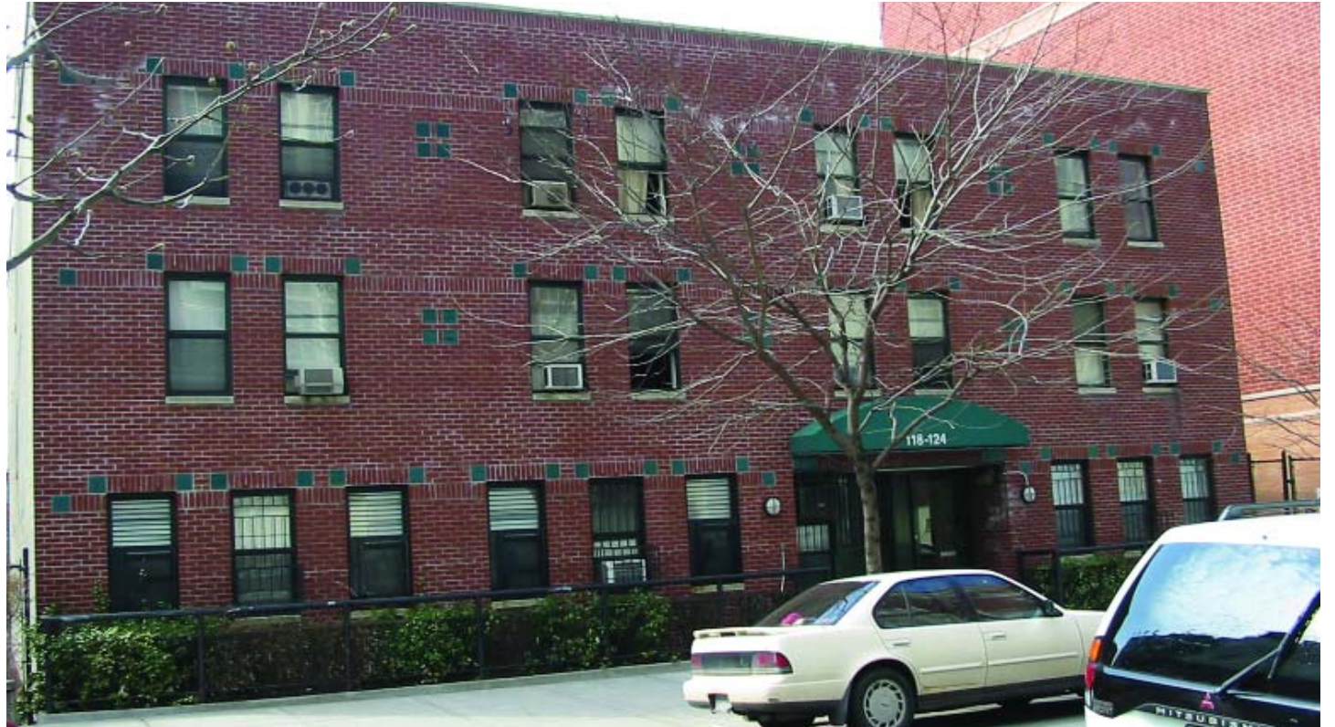
Bridge House 8, pictured above, provides 20 units of housing for formerly homeless, mentally ill adults in East Harlem. The building and program design will serve as the prototype for new housing to be constructed with the support of the Deutsche Bank SHARE program award.
