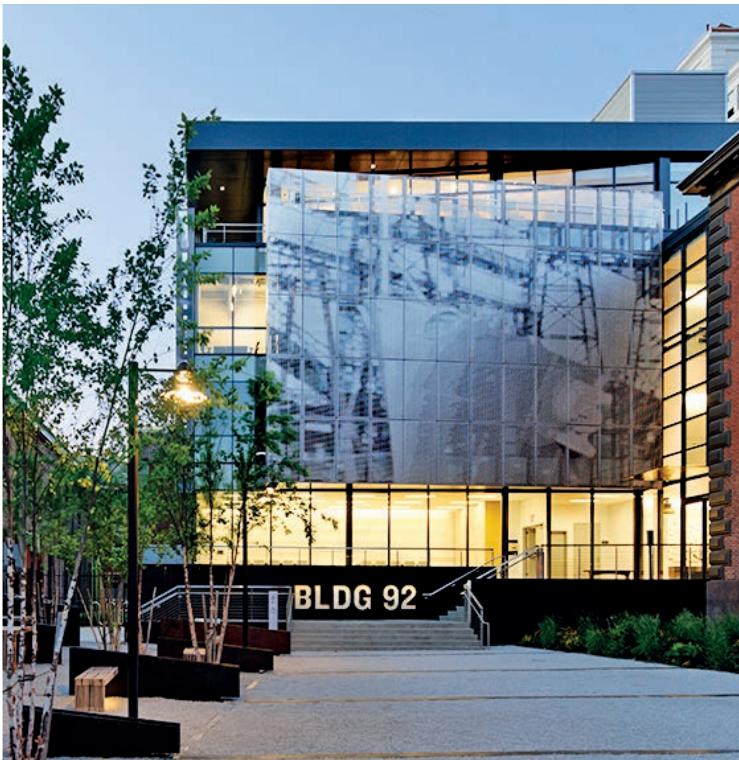
Building 92 is the Yard's employment, exhibition and visitor center. The Commons will provide a café and event space open to tenants and the public, strengthening the Yard's unique bonds with the local community Photograph by Chuck Coi, courtesy BNYDC
